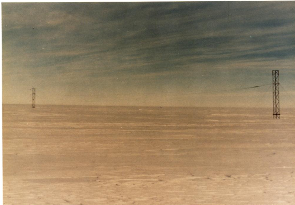
MCMURDO AREA OF THE ANTARCTIC. The antenna are 120 feet tall, built during the 1965-68 period. Approximately 15 feet of the towers are now showing, which means four to five feet of ice increase per year average. (SEE MAP BELOW)
